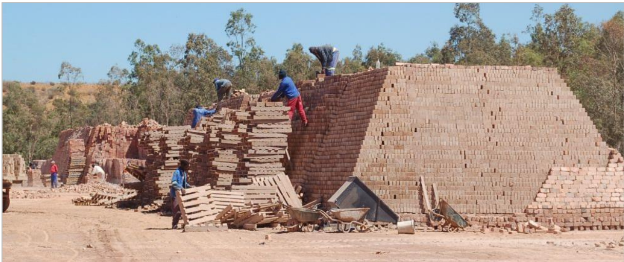
Figure 1: Open air clamp kiln. Source: Worcester Brick
