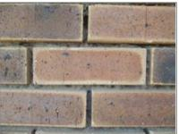
The extent of surface weathering of the face bricks was estimated at 2-3% which is relatively low considering the extreme sea spray conditions.
